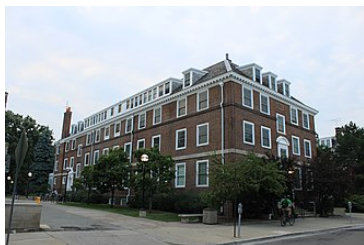
Betsy Barbour Residence Hall , one of three all-female residence halls on campus, was designed by Albert Kahn in the English Georgian style .
