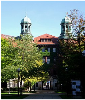
West Hall at the Southeast corner of the Diag
